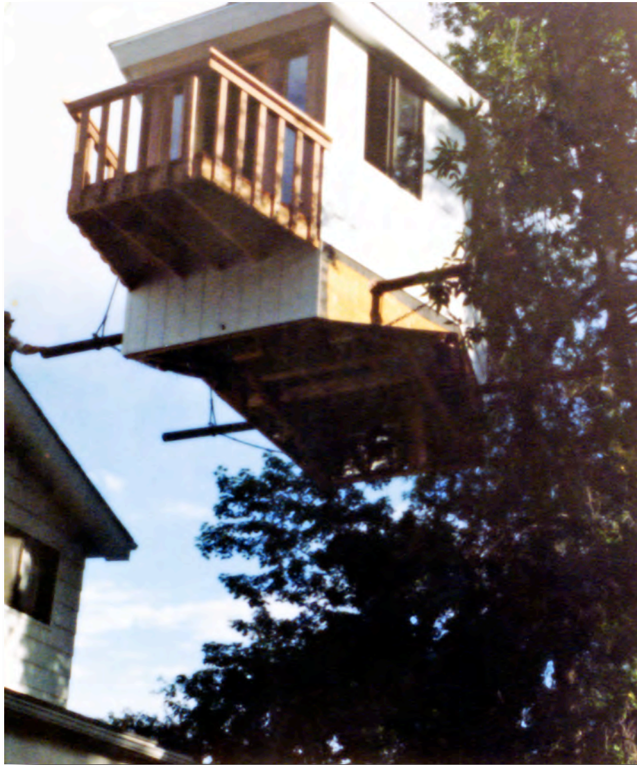
FAR OUT project, built at the wood shop and crane set on top the house across town.
