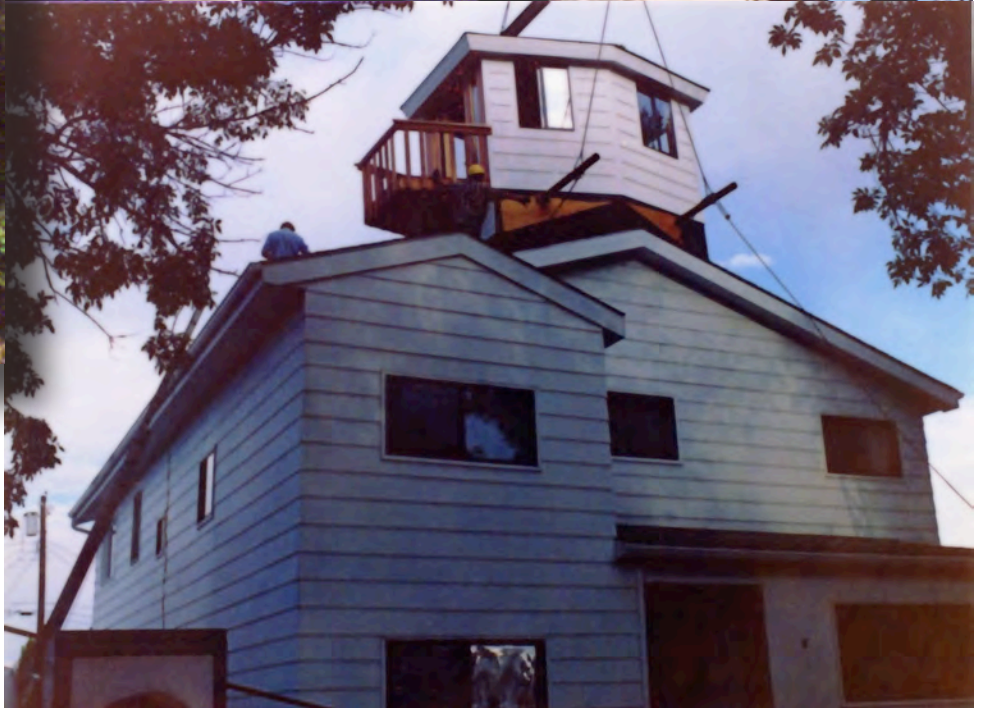
FAR OUT project, built at the wood shop and crane set on top the house across town.
