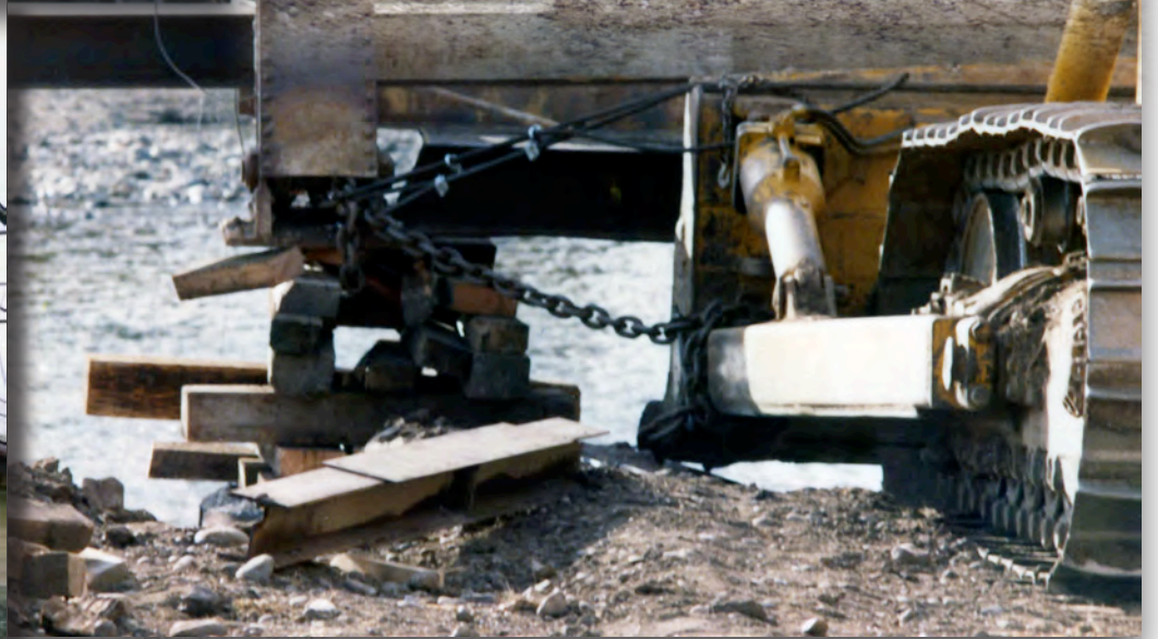
Making ready to pull through the river.
