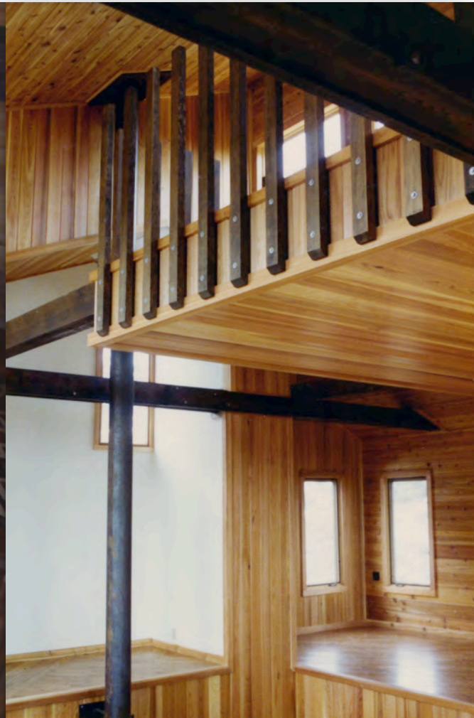
The old log 'dug-out' below the nice wood floor of the new building from the second floor up.
