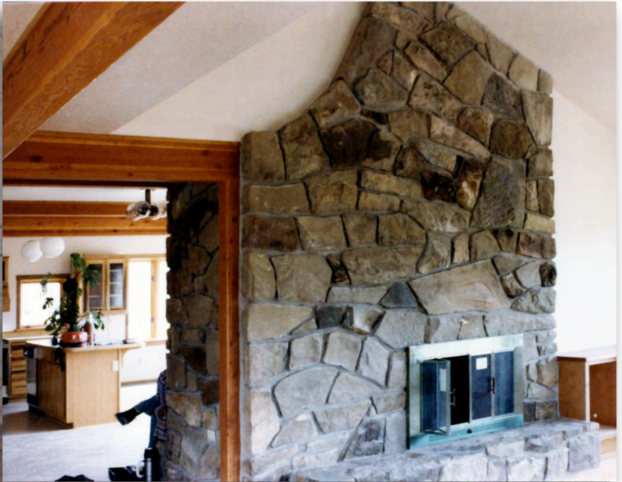
One of two fire places back to back.
