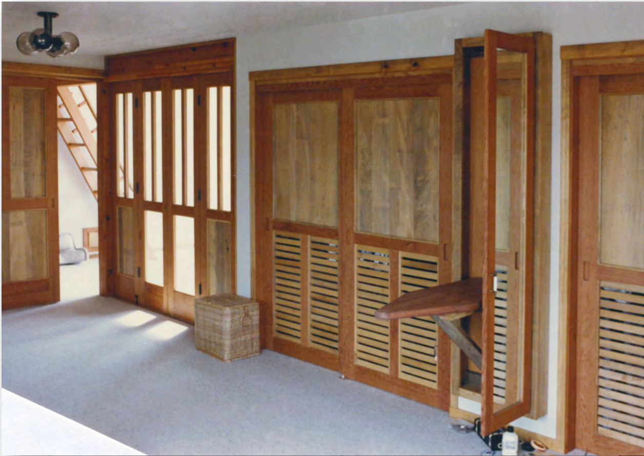
Master bedroom closet and entry door set. Ship's ladder to loft storage cabinets and air return for solar heat gain recirculation.
