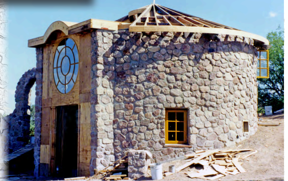
Southwest and South east elevations under construction.
